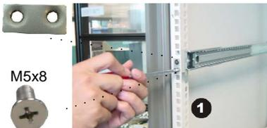
Screw the rails onto the rack.
